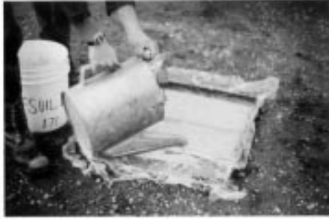
FIG. 4 Sand Being Poured Into the Template
